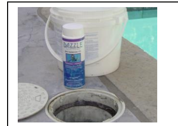
Dazzle™ Pro Balance UV Mix in pail of water to form slurry and slowly pour into clean skimmer.
